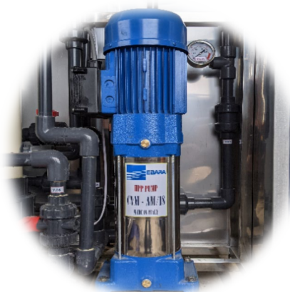
BƠM LỌC CVM – ITALY ( CVM filter pump – Italy )
